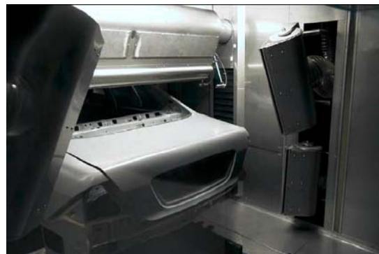
Nozzles at the side station and roof station
